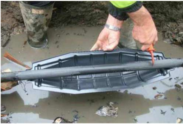
Fig.9: The joint installation beside permanent water source [16].
